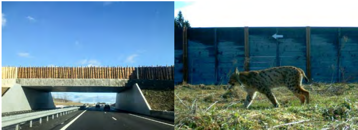
Example of a wildlife crossing over a divided highway (© OFB/S. Gatti). These wildlife crossings can be used by lynx. Suitable fencing must be provided to direct them towards these structures so that they can get across any obstacles safely, here in the Doubs (© FDC25).
